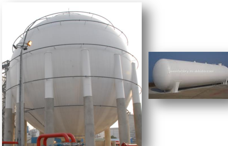
Figure 6. Examples of spherical and bullet LPG storage
